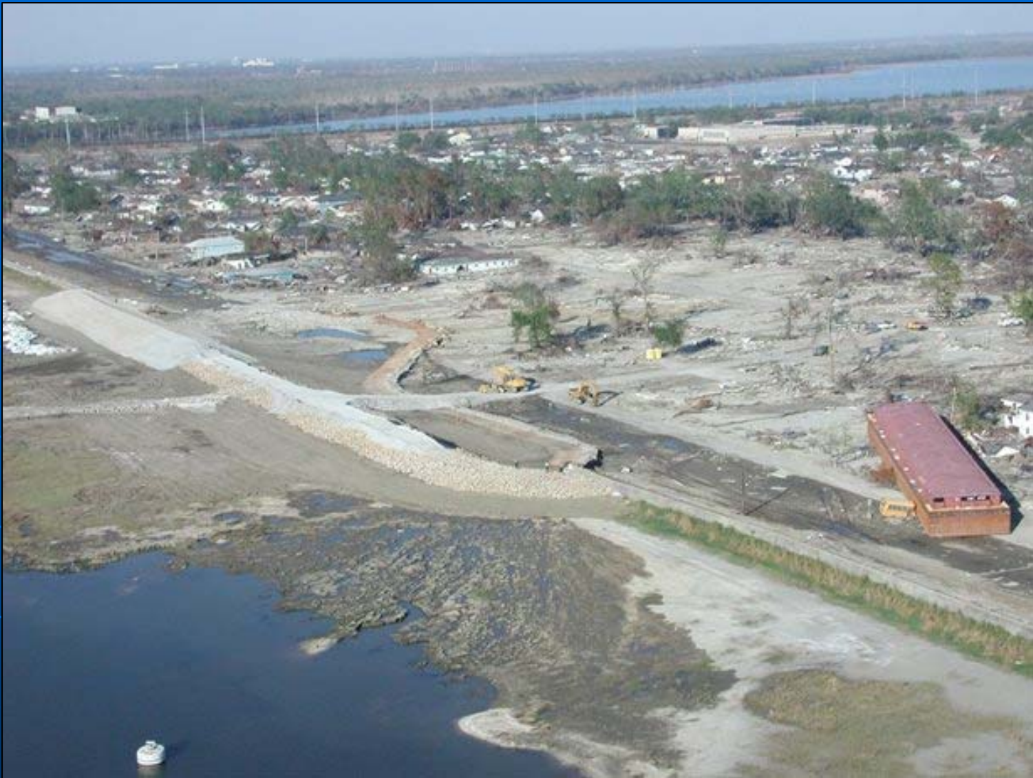
Aerial view of the south breach at the east bank of the IHNC (at the west end of the Ninth Ward), showing the 'wet spot' along the inboard side and the crevasse splay generated by reverse drainage flow. [Photograph by U.S. Army Corps of Engineers]
